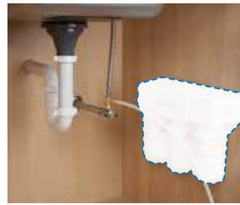
**6** Unit Installation: Select a space under your sink for the filter unit that is at least 12 inches from the bottom of your cabinet and allows for easy access to your cold water supply and for filter replacements. Use the mounting holes located at the back of the unit to mark the wall screw placements with a pencil. Center to center hole distances:
