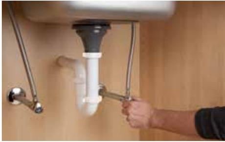
**1** Unpack and unwrap contents. Turn off and disconnect the cold water supply.
