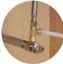
**4** Faucet Installation: Install as shown. Tighten nut to secure faucet to sink.
