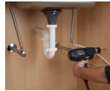
**7** Use a 7/32" drill bit to drill holes for the plastic anchors provided. Carefully tap the anchors into the drilled hole with a hammer. Mount unit to the wall with the screws. For the AQ-5200 and AQ-5300 — Pull the protective plastic strip from the battery compartment. The red LED should flash and beep five (5) times to indicate that the battery is installed correctly.
