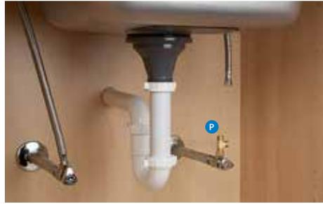
**2** Attach threaded ends of supplied brass tee to the cold water supply line and shut-off valve; tighten using an adjustable wrench.
