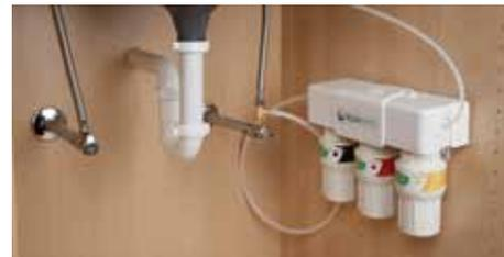
**10** Turn the cold water on. Check for leaks and proper installation: place a towel under the filter unit and check for leaks. Allow water to run for 10 minutes to flush carbon fines. Note: Never use oils to lubricate the O-rings; O-rings come pre-lubricated.
