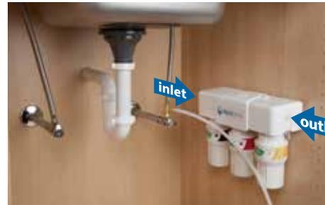
**9** Connect supply lines: insert tubing from the tee fitting into the inlet side and insert tubing from the faucet into the outlet side. Use diagram on the right to mark tubing depth to ensure they get inserted completely. **It is VERY IMPORTANT to insert tubing completely so leaking does not occur.**
